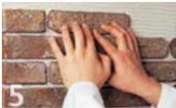
Then apply the brick strips in a sliding motion. Always start with the corners and mix strips from different boxes.
