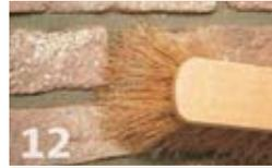
Clean away the extra mortar with a stiff dry brush before it has completely dried.
