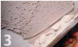
Apply the adhesive in sections of 0.5 m<sup>2</sup> so it doesn't dry before you fix the brick slips. It is best to work going down, avoiding stains from spotting and spilling.
