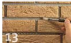
Interfix joints can be filled in the traditional manner. Or the Interfix glue can be stroked smooth in the joint. Do this with a damp finishing brush, such that the glue seals with the edge of the strip.
