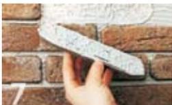
In this way you can monitor whether the strips are firmly fixed to the wall.
