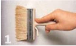
The surface must be consistent, flat and clean. It must be dry and free of grease. If the surface is porous then apply first a layer of Cemix Primer. Allow to dry for 2 hours then you can begin.
