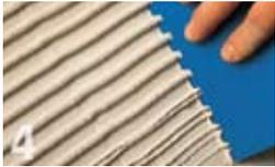
Start by making ribs in the glue with a notched spatula (6 mm for interFix, 8 mm for Granulit and 10 mm for Murok and Interock).
