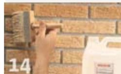
Outside walls should always be sealed with Silifin. The wall must be completely dry before you apply the Silifin with a brush until thoroughly covered.
