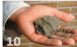
Filling joints is done with Cemix Unijoint which is mixed with water. In the right proportion the mix is still a bit rough, sticky and on the dry side. Keep using the same proportion of water to avoid colour variations.
