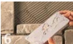
For the heavier stone products of the series (Murok and Interock) installation with the buttering-float technique is necessary. This means that the glue must be applied on the back of the slips as well as on the wall surface.
