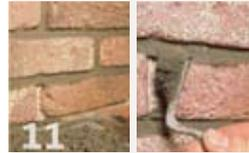
Apply the joint-filling mortar with a traditional pointing trowel and sweep clean with one stroke. The vertical joints are usually a bit smaller than the horizontal joints.
