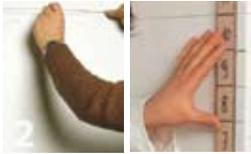
Section off the wall in areas for about five brick strips. Allow 1 cm for the joint. Within these sections you can work by sight.
